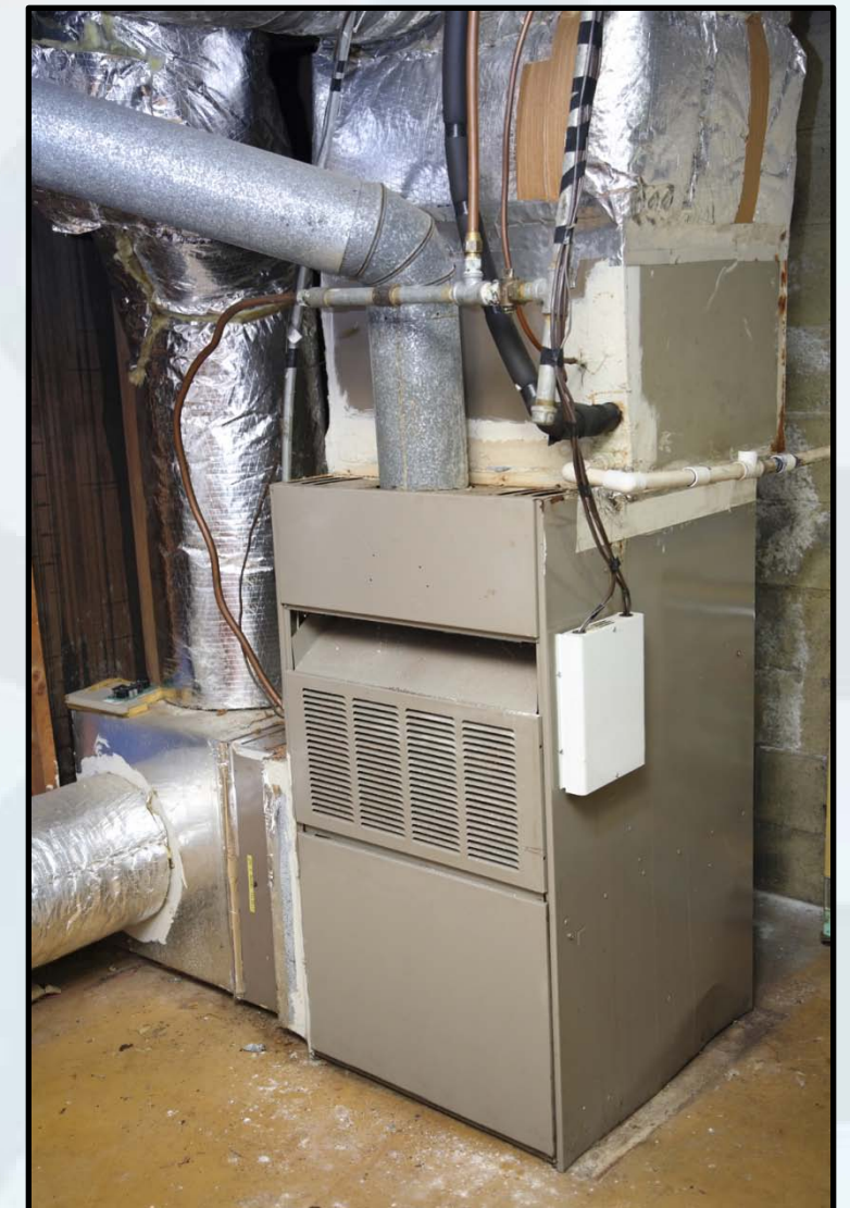
Typical Home Heating/Cooling System
