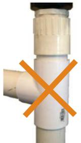
Avoid the use of a tee within the stand pipe. A tee can create false signals which will interfere with the sensor's performance.
